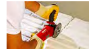
3- Cutting the panel by angle-grander
