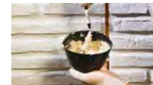
6- Preparing the assembly putty
