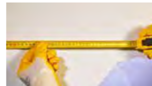
1- Measuring the application area
